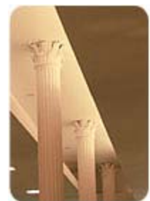
Intumescent fireproofing applied to ornamental columns at Bloomindales Soho.
