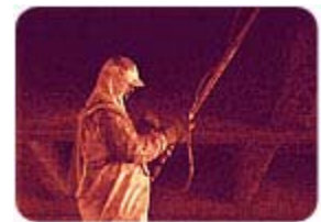
Sprayer at the PATH Terminal Restoration Site, at Ground Zero.
