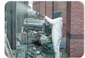
Spraying mineral fiber fireproofing at the Highlands Project, in Brewster, N.Y.
